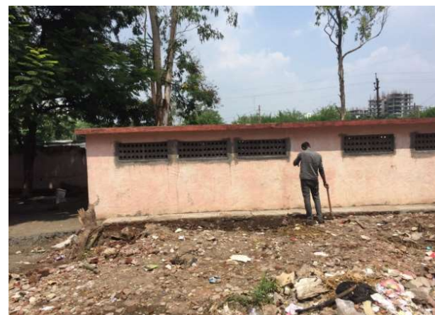
now (Paving work will be done here)
