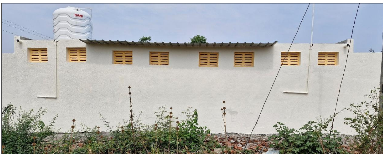
CONSTRUCTION OF SANITATION UNIT
