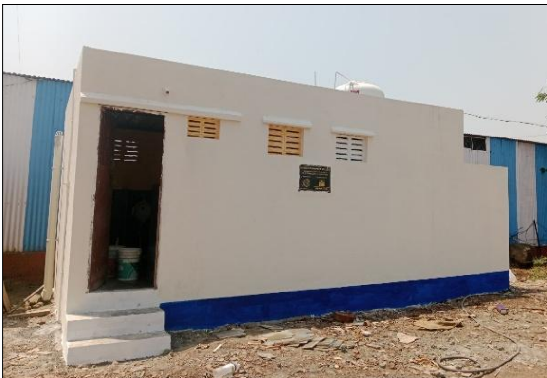
SCHOOL- 8 – NEW ENGLISH SCHOOL, ANGAPUR, SATARA CONSTRUCTION OF SANITATION UNIT
